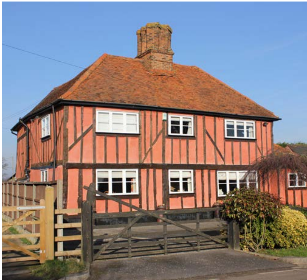
Figure 12. Grade II Listed Wells Farmhouse
