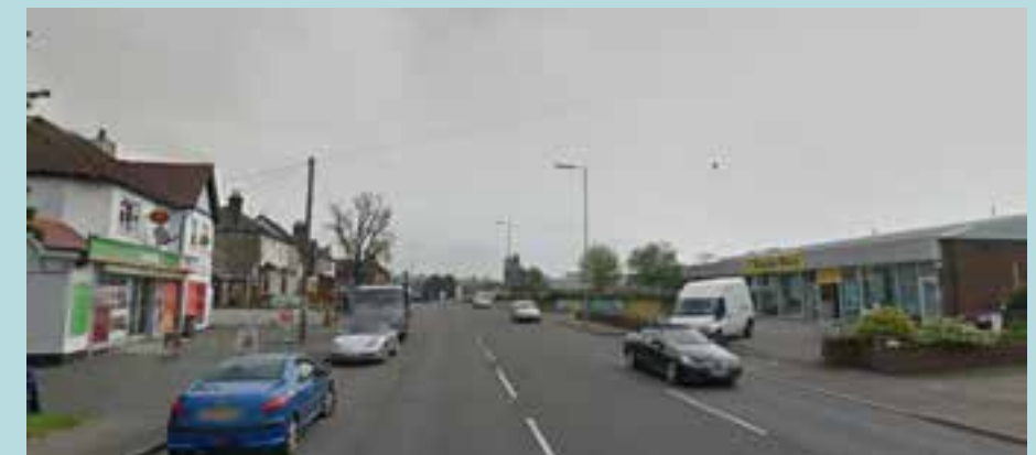
Londis & post office, and Topps Tiles
