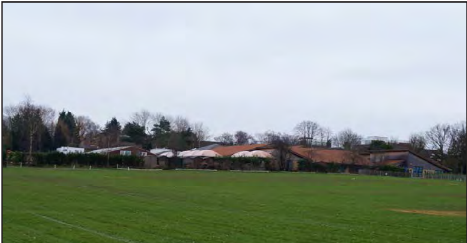
Primary School buildings lying to the south of the site.
