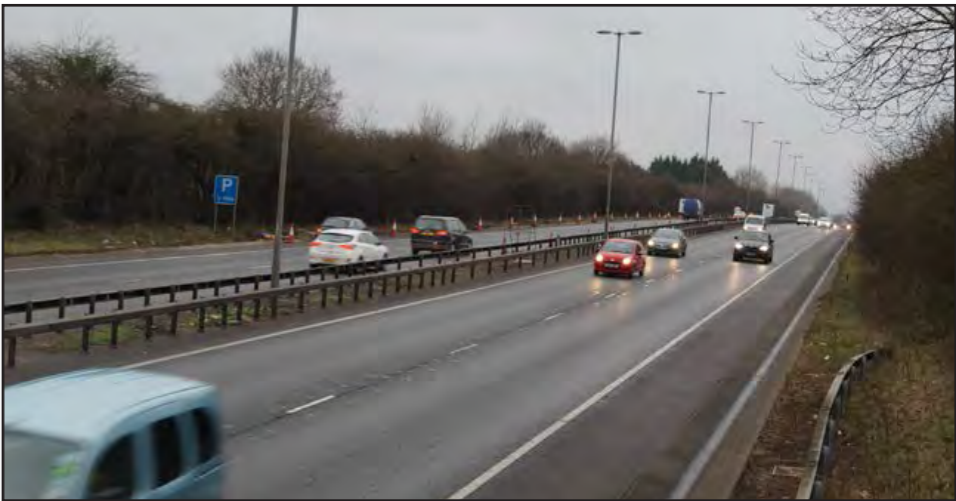
A12 Dual Carriageway
