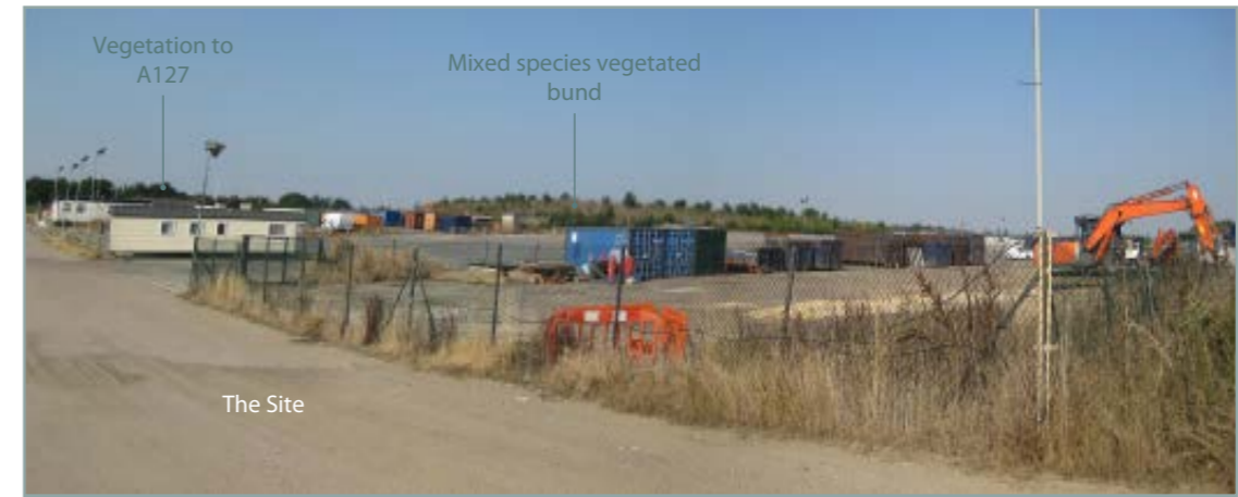
Photograph P1.4: View north-northeast over the Site from watercourse crossing
