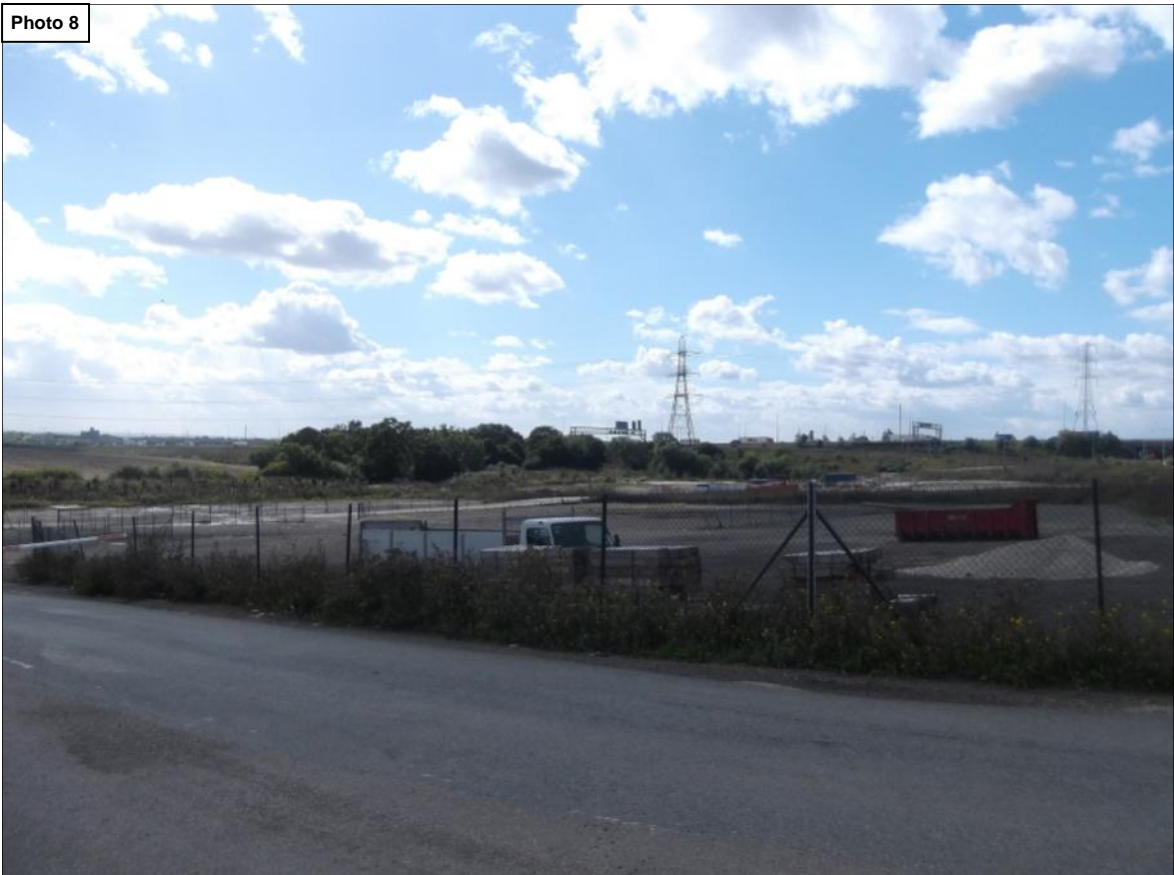
View of the depot section of the site
