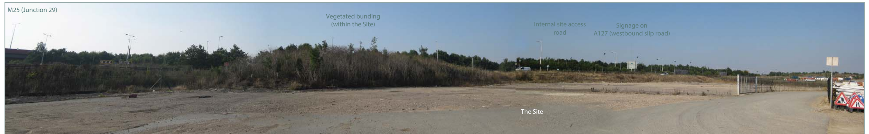
Panoramic Photograph 18: View north-east towards M25 (Junction 29) and A127
