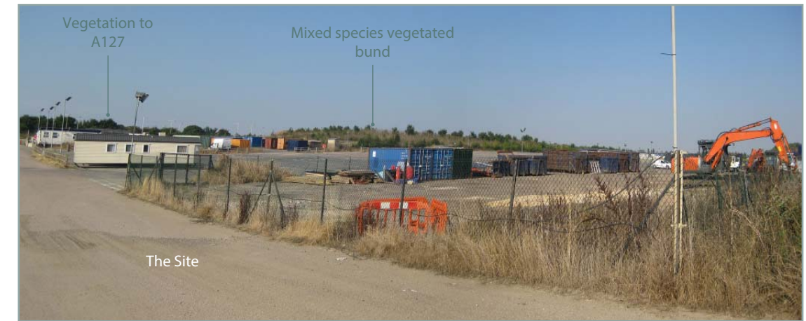
Panoramic Photograph 24: View north-northeast over the Site from watercourse crossing
