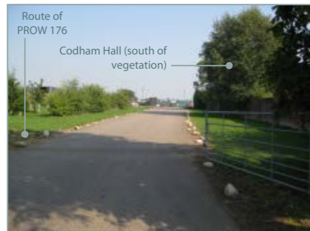
Photograph P4.2: View east to eastern compound areas
