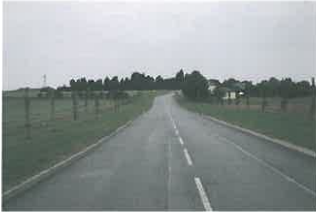
Access road from A127
