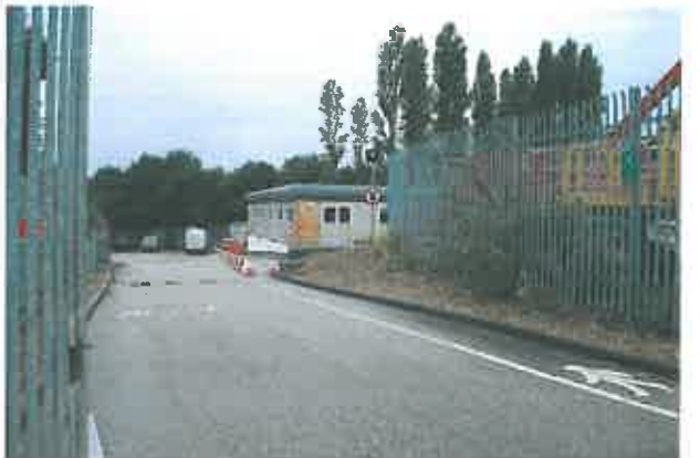
36, Entrance to ECC highway depot
