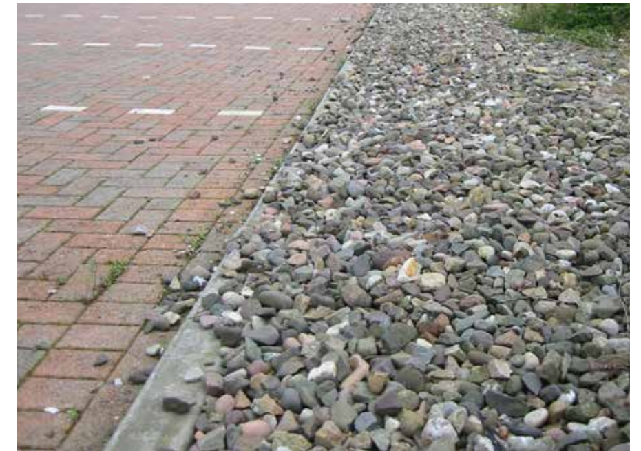
Mixture of permeable paving surfaces
