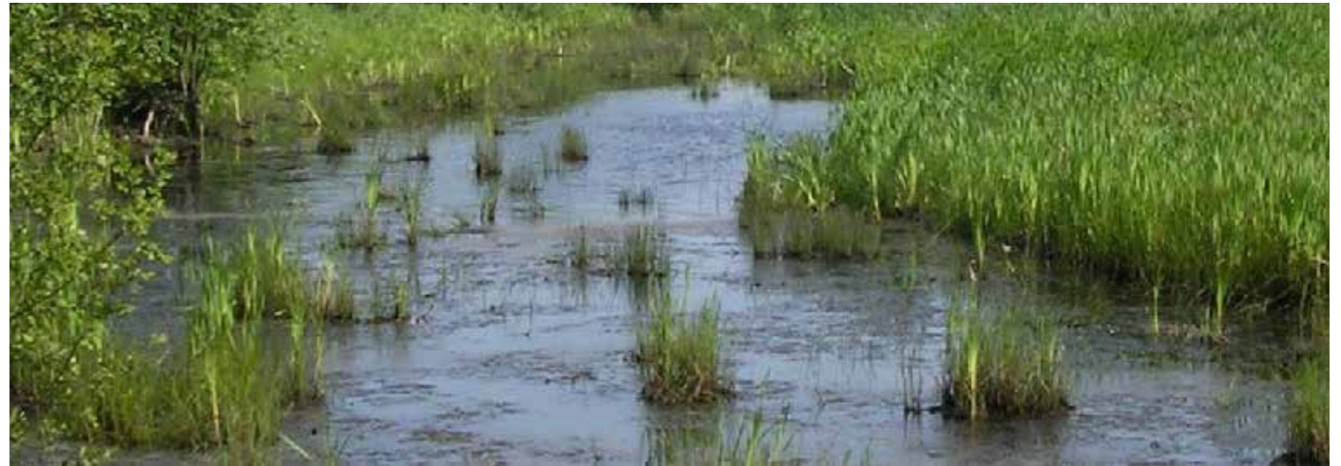
Drainage attenuation ponds
