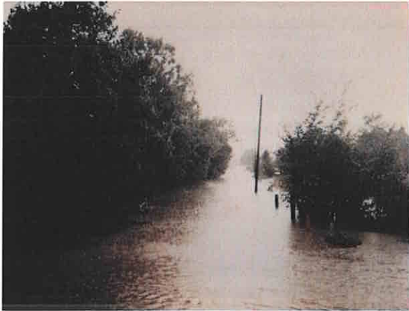
Above: Chelmsford Road flooding - 1987 The River Wid
