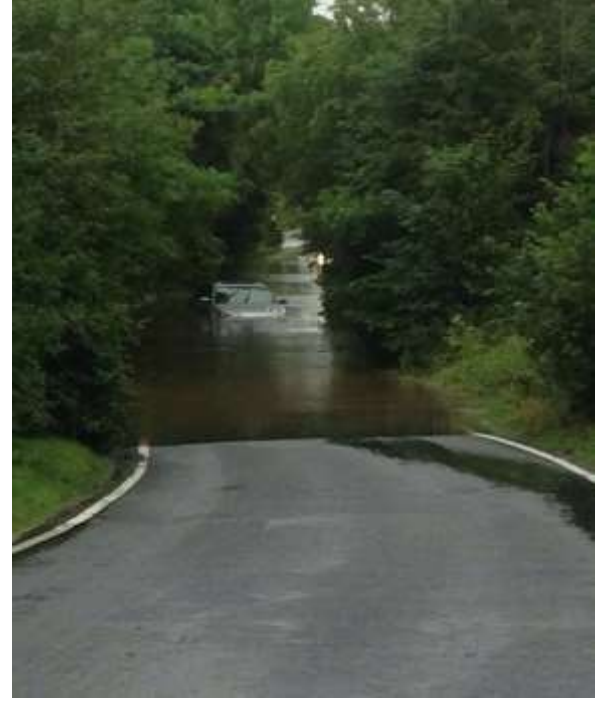
Above: Flooding on Redrose Lane - 2016 (note depth of water)
