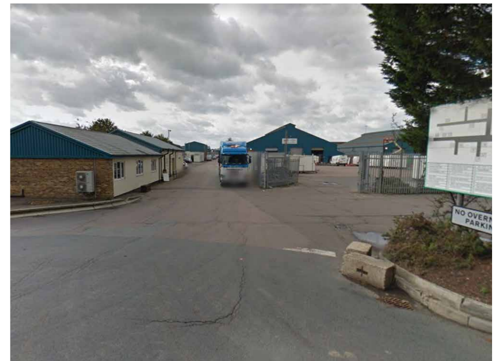
View F from site entrance. This view shows the estate office and larger units in the background.
