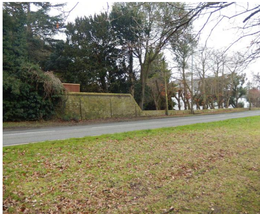
Boundary walls along the frontage at Hutton Court (formerly Hutton Park) iv
