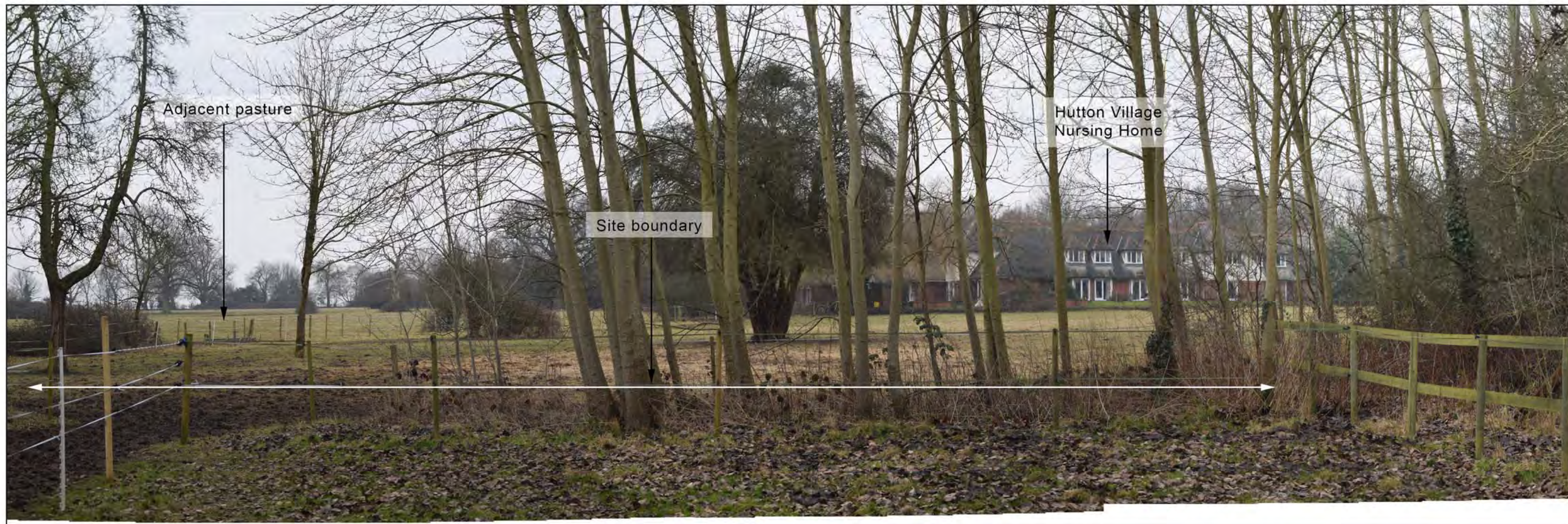
Location: View of southern Site Boundary.
