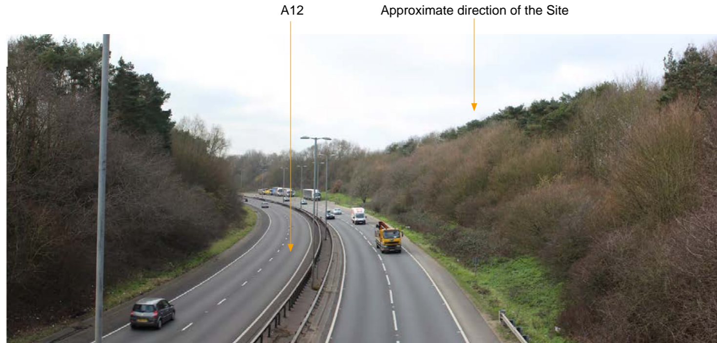
PHOTO VIEWPOINT D: VIEW WEST FROM ONGAR ROAD BRIDGE OVER A12
