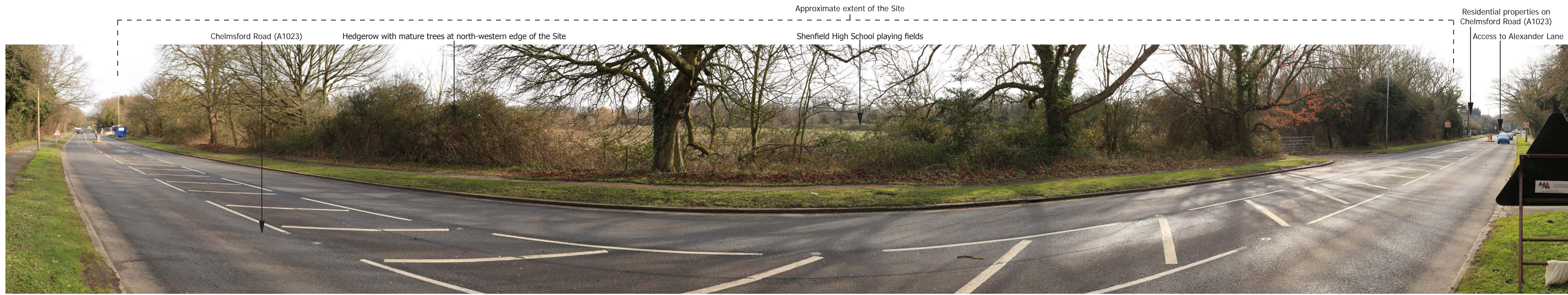
SITE CONTEXT PHOTOGRAPH 4: VIEW SOUTH-EAST FROM CHELMSFORD ROAD
