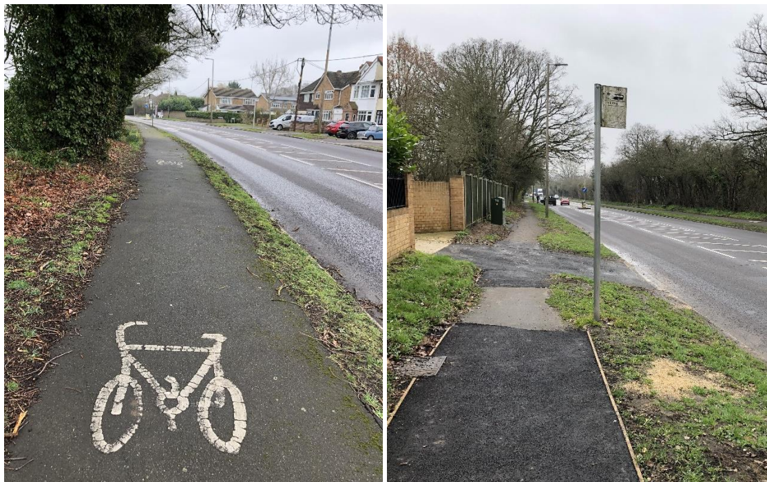
Image 3.1: Left: dedicated cycle route on the northern side of the A1023 Chelmsford Road; Right: Footway of the southern side of the A1023 Chelmsford Road
