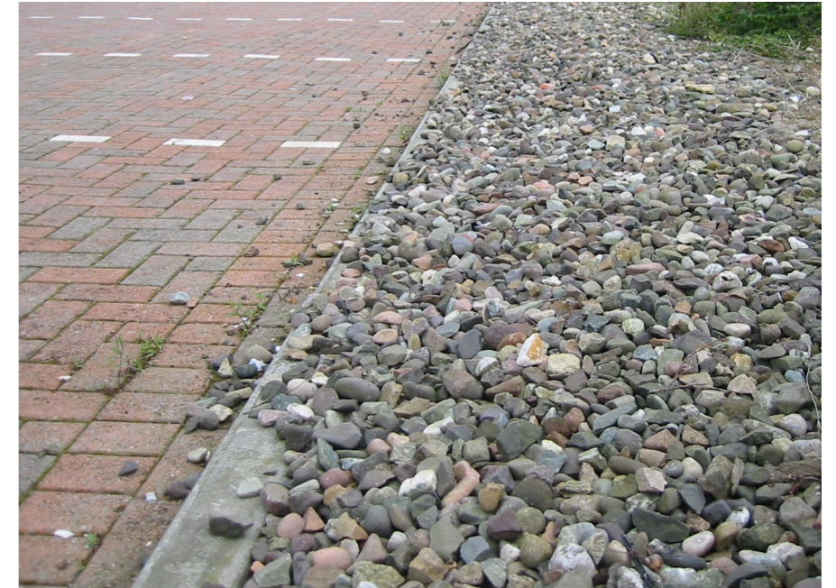
Mixture of permeable paving surfaces
