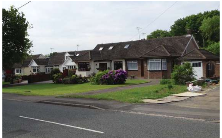
Bungalows situated together along Wyatts Green Road
