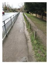
Sections of the footway in the vicinity of the schools requires upgrading and widening to accommodate the level of pedestrian movements in this area; routes across grassed areas, indicated by wear, demonstrate that the existing footway does not provide sufficient width (left).
