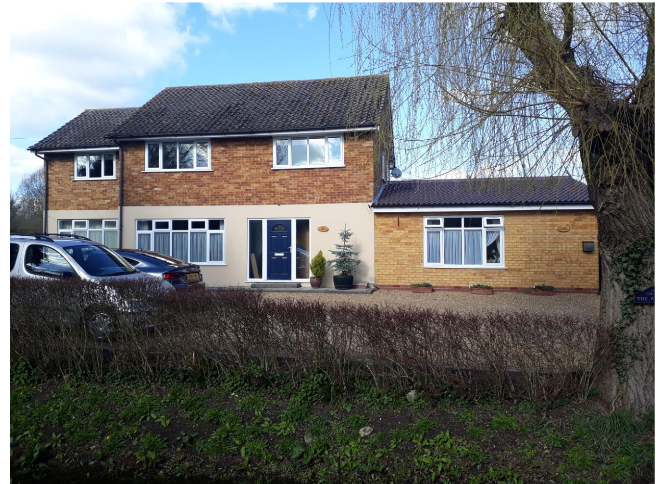
Figure 4.7 – Residential development to the west of Wells farmhouse
