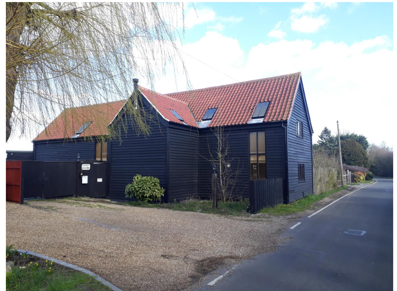
Figure 4.2 – Adjoining barn conversion
