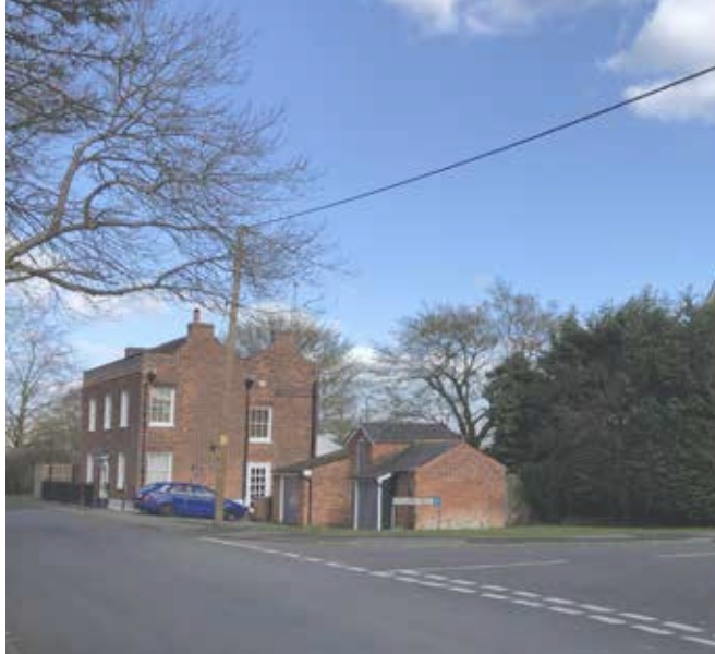
Figure 27. Grade II Listed Woodbines
