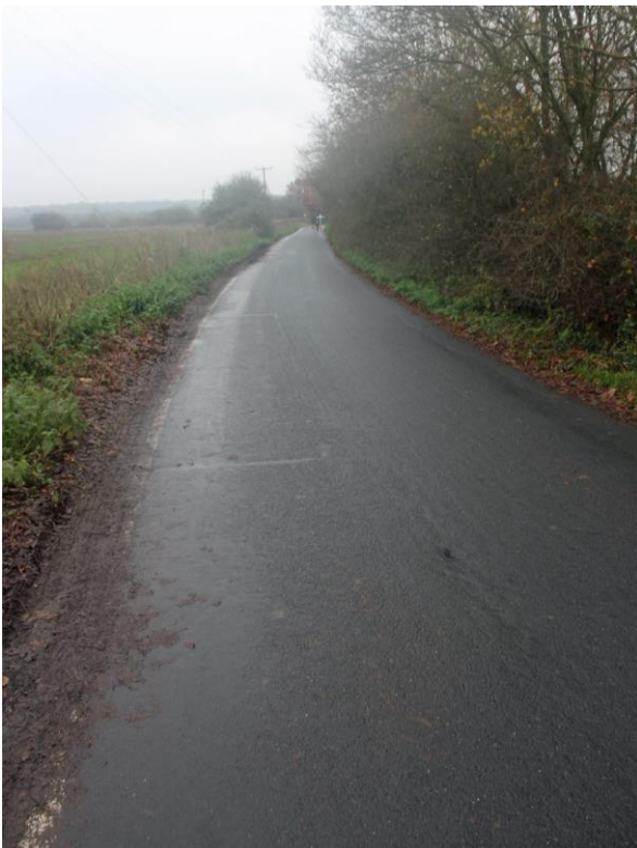
Further image of Redrose Lane - note cut-up verges and lack of centre lines (i.e. delineating insufficient width for two vehicles to pass)
