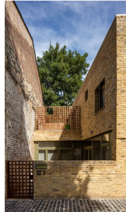
Peter Barber Architects, Moray Mews houses
