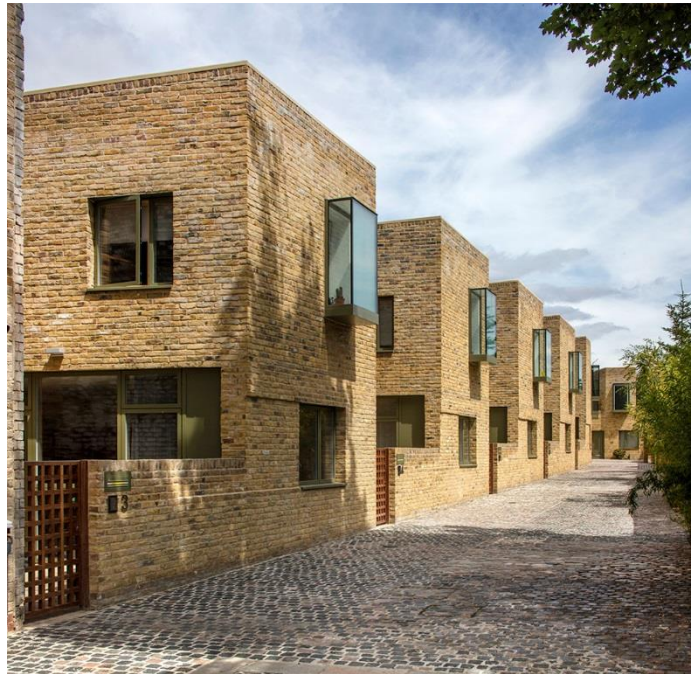
Peter Barber Architects, Moray Mews houses
