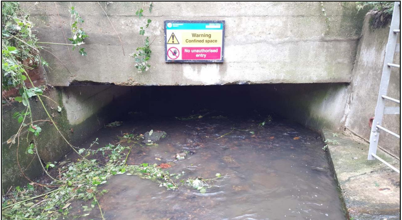
Figure 10: Culvert beneath Spital Lane (Source: BB Surveys Ltd, August 2015)
