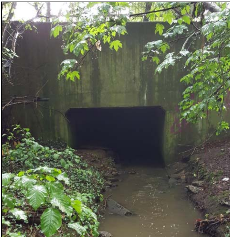
Figure 11: Culvert beneath Spital Lane/footpath (Source: BB Surveys Ltd, August 2015)
