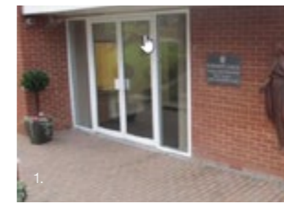
Figure 5.3B - St. Helen's Catholic Primary School
