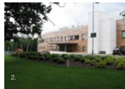
Figure 5.2C - Brentwood Community Hospital
