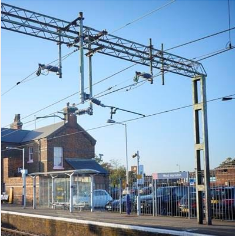
Station Approach, West Horndon, Brentwood, Essex
