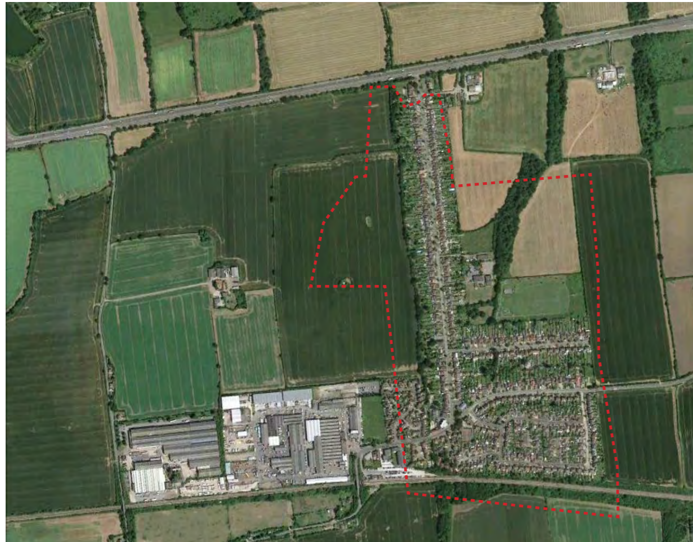
West Horndon aerial photo (courtesy of Google Earth 2013)
