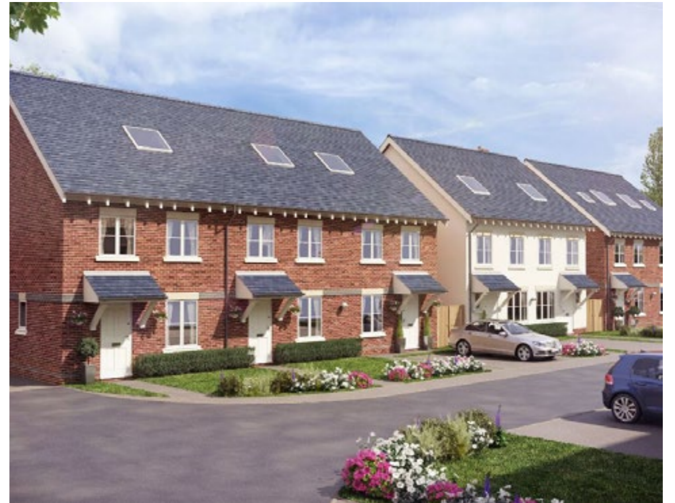
Figure 6.1C - Kenton Lane, Harrow
