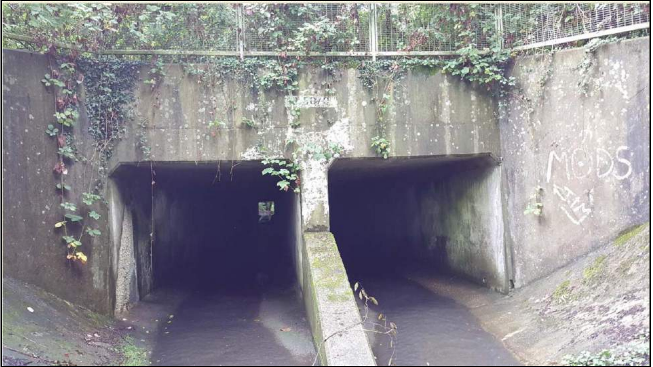
Figure 12: Twin box culvert beneath Wigley Bush Lane (Source: BB Surveys Ltd, August 2015)
