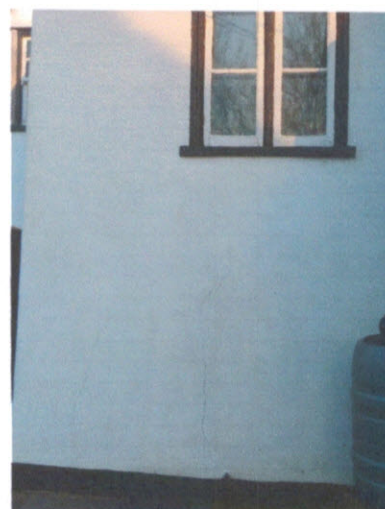
Cement render on stair tower
