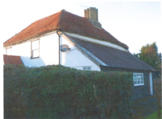
Central six-shafted chimney stack
