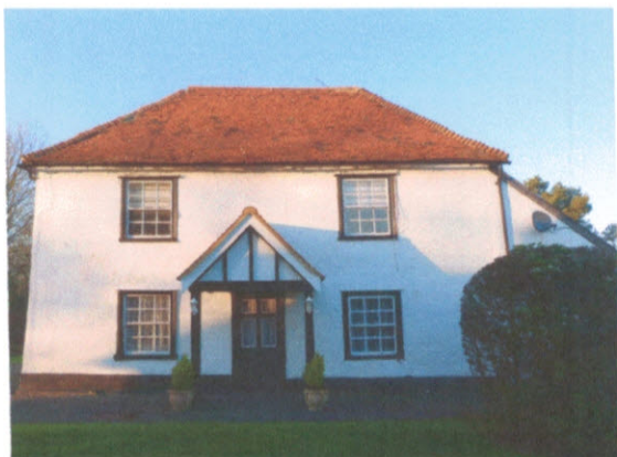
South elevation with porch and 18 th century sash windows
