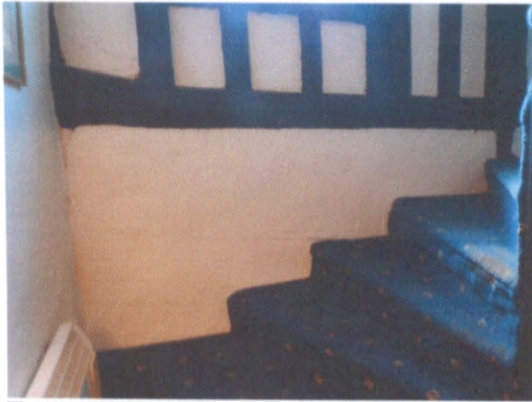
Typical black-painted timbers in stair tower
