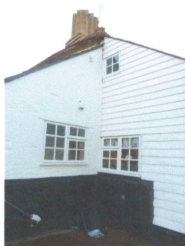
20 th century windows to be repaired or replaced
