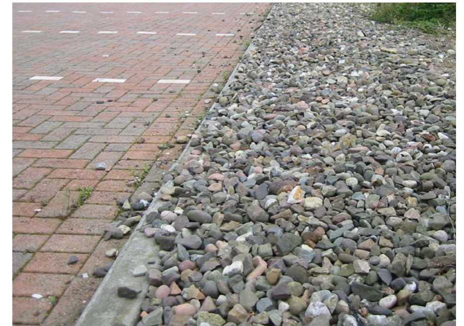
Mixture of permeable paving surfaces
