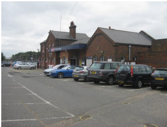
The Station entrance
