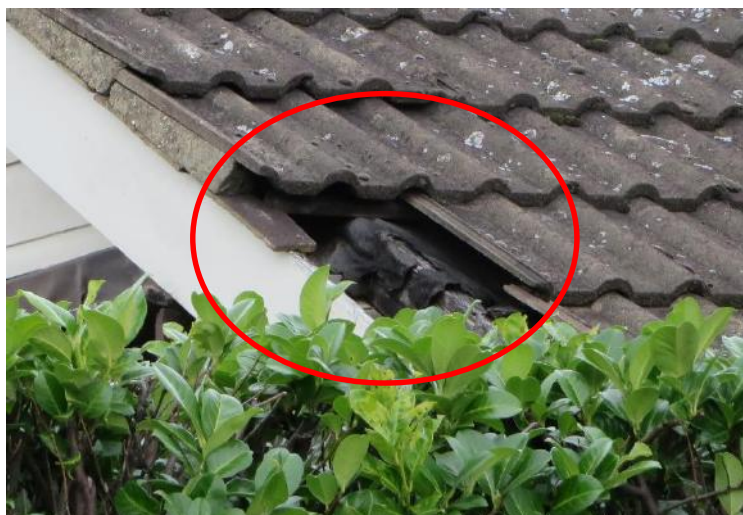
Photo 12 – Missing Tile on Building 2
