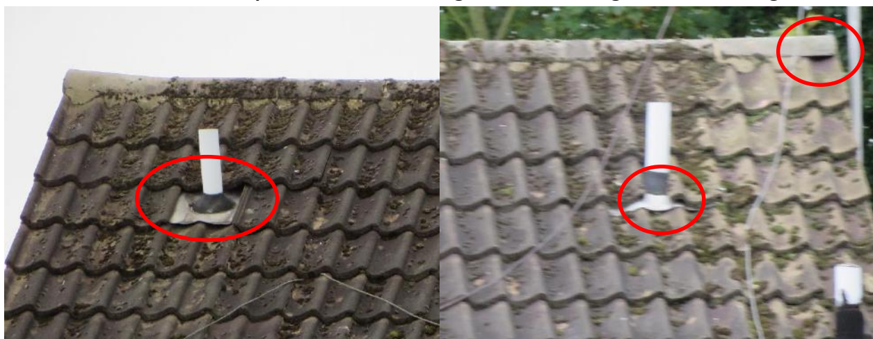
Photo 9 & 10 – Gaps under Lead Flashing and Central Ridge Tile on Building 1
