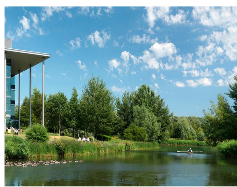
HIGH QUALITY WATER FEATURE WHICH ACTS AS A RAINFALL OVERFLOW AS WELL AS PROVIDING VISUAL AMENITY TO THE PARK
