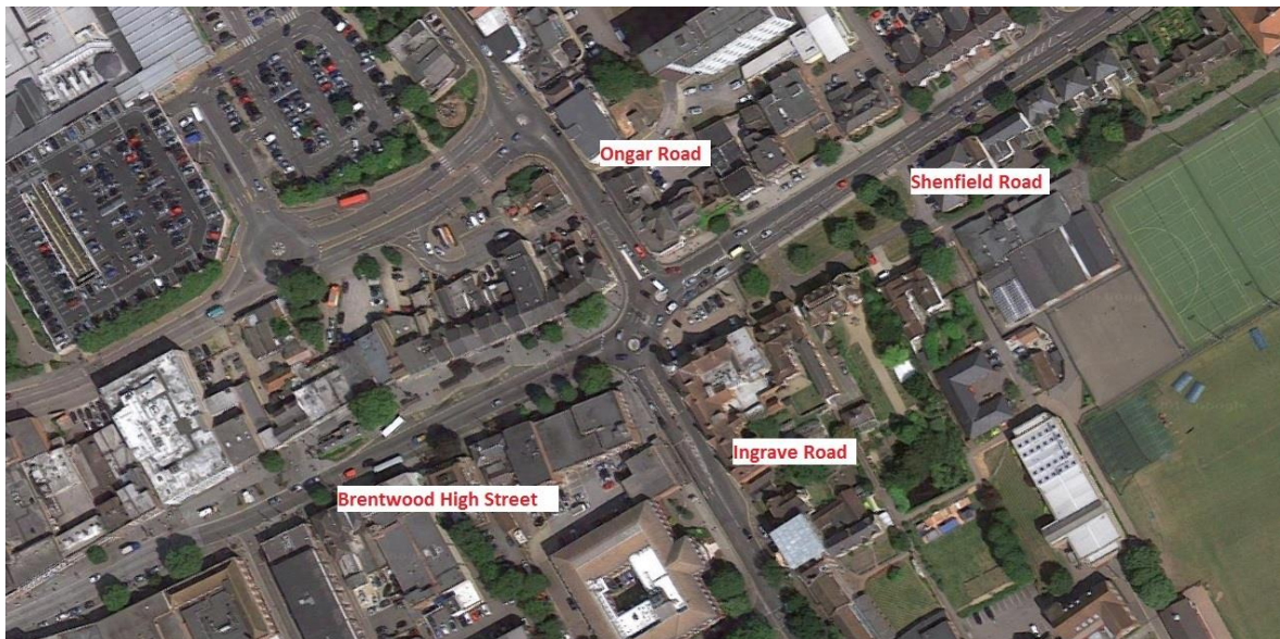
Figure 1: Aerial view of the Wilson's Corner Junction
