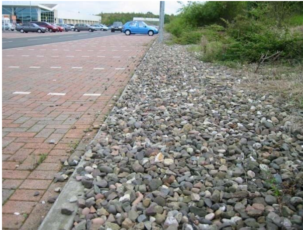
Figure 4a: Permeable paving.
