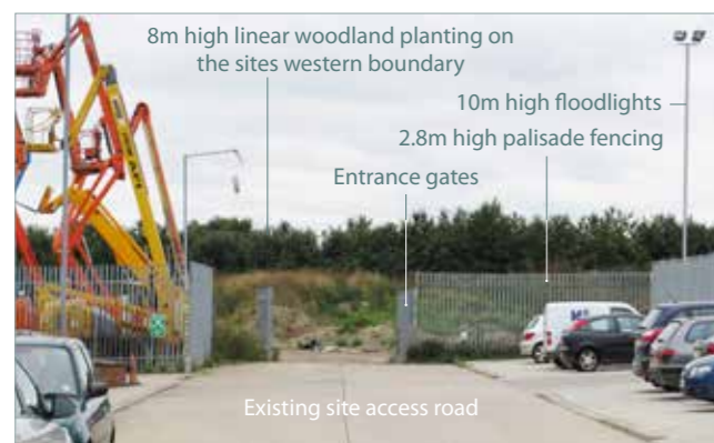
Image 8: Looking west towards the palisade entrance gates into the Site
